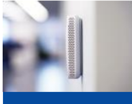
Indoor CO 2 CO 2 sensor on the wall, ideally 1m from doors, windows & vents, around breathing height.
